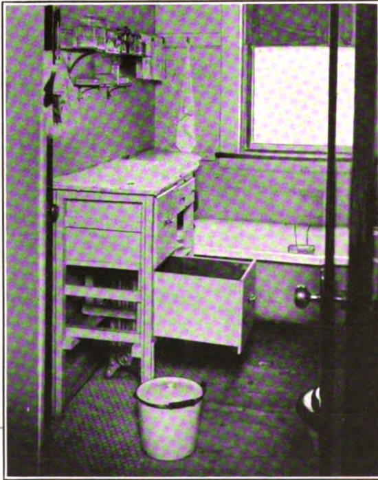
FIG. 92.—Special bath room equipment for private home, showing dressing table (padded) with drawers, built over radiator. Shelves for dressing, etc., above the table. Bathing board over one end of bath tub.
